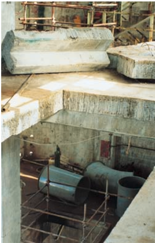
Partial demolition of heavily reinforced concrete ceilings
