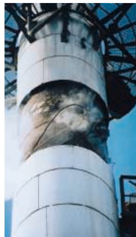
Demolition of double-walled steel structures
