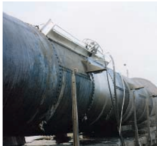
Cutting openings in large storage vessels
