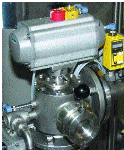
Example of T-Port Valve equipped with Sliding Couplings utilised as a Launching and Receiving Station.
