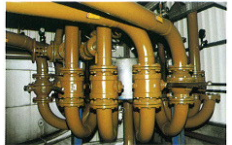
I.S.T. rotary manifold: a group of tanks used in the lubricating oil industry are linked with the I.S.T. rotary manifold.
