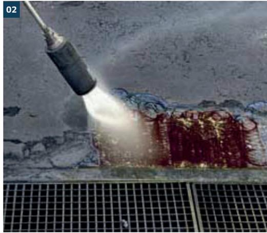
**01** Equipped with up to 3000 bar, the removal of stubborn concrete is possible.
