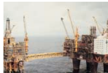
Oseberg Twin-Platform in the North Sea WOMA Ecomaster has been used here successfully for surface preparation and derusting of steel surfaces
