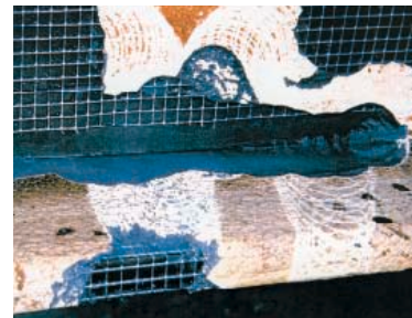
Removal of heavy intumescent coatings with hand-held water jet tools
