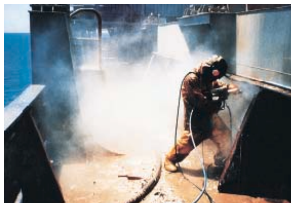
Derusting and decoating of steel surfaces using a water jet tool
