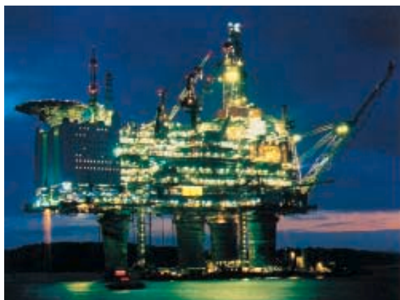
Gullfaks Gas and Oilfield At the platforms A and B, several WOMA Ecomaster systems are used successfully for surface preparation, pipeline maintenance and tank cleaning
