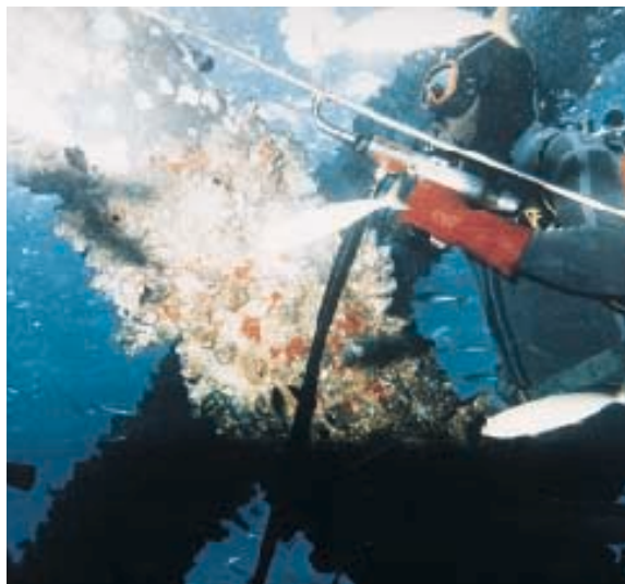
Submerged cleaning using a reaction force reduced underwater tool
